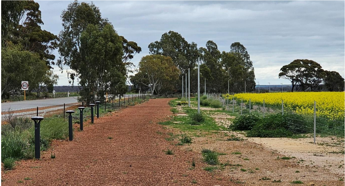
Figure 4: Street view photo existing constructed foot path
