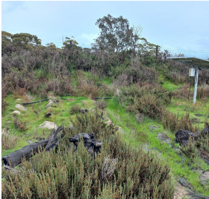
Photo B-2: Pond outer bank showing potential seepage and established vegetation
