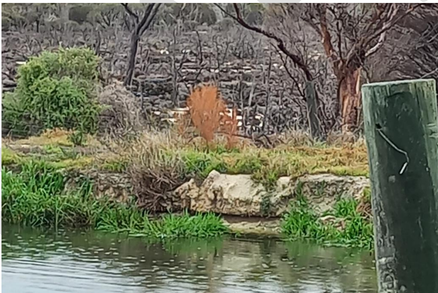
Photo B-5: Evidence of damage to internal pond banks from wind-driven wave action
