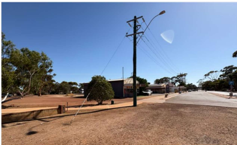
Figure 2: Existing Western Power Uni-pillar & Overhead WPC services along Marshall St.
