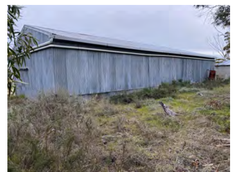
EXISTING BUILDING PHOTOS
