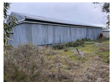
EXISTING BUILDING PHOTOS
