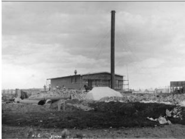
The Ghooli Pumping Station in 1902, shortly before it began operating. (Supplied: State Library of Western Australia)
