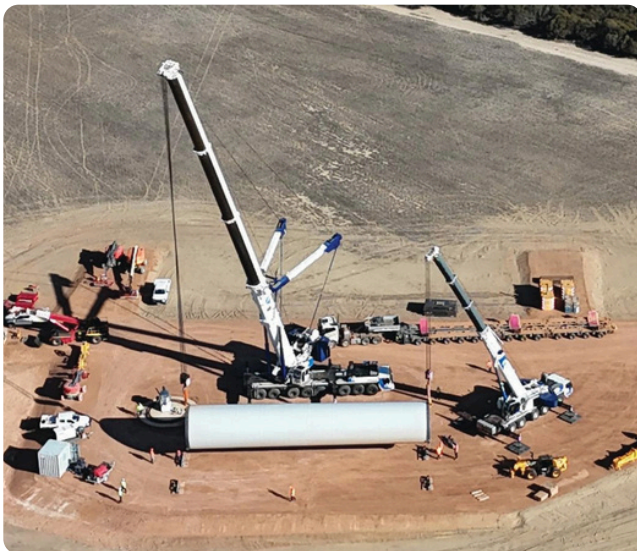
TURBINE TOWER SECTION BEING LIFTED INTO PLACE.
